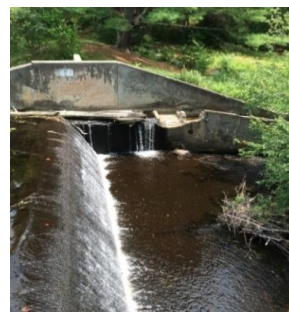
Breakheart Pond Dam
